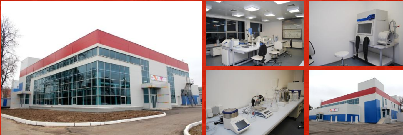
THE PHARMACEUTICAL MODULE IN THE TERRITORY OF TECHNOLIS "HIMGRAD"
